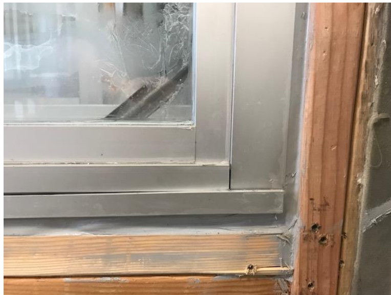
Photo No. 2 Detail photo of corner of AP-25 Installed
